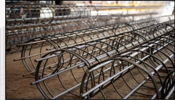
Pre-fabricated Cage (Bored Pile Cage)
