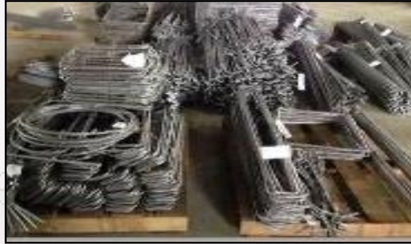
Rebar Cut and Bend
